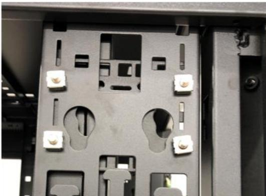
Top PDU bracket cage nuts
