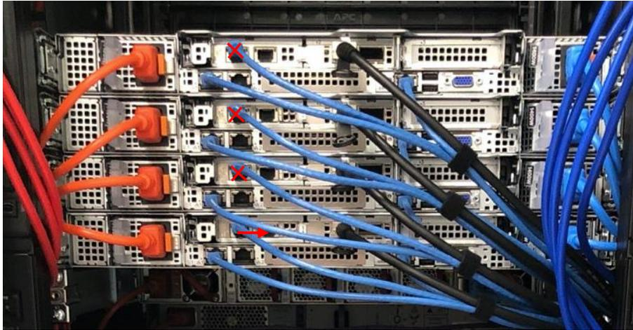
Note that the photo above shows the four-server version. The default build has one server (the one in the lowest position).
